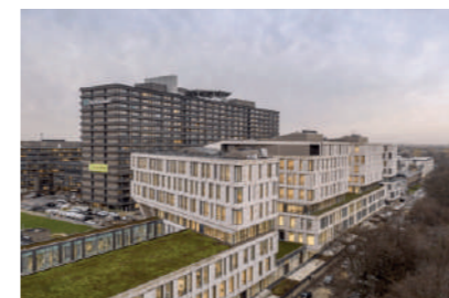
Rigshospitalet / Copenhagen - Danimarca
